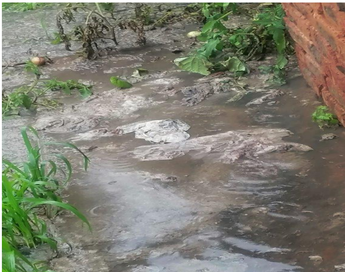
Figure 1 : Raw sewage material forming a large puddle in the Complainant's yard.
