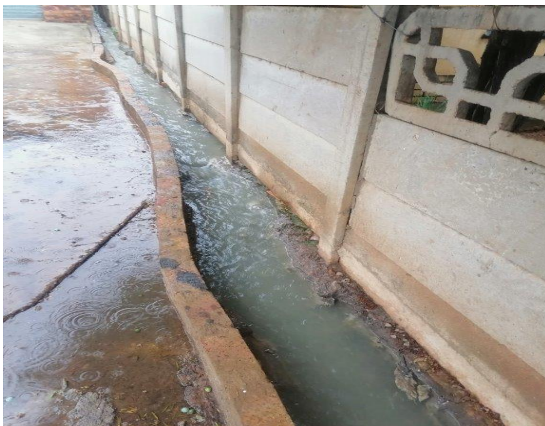
Figure 2: Raw sewage flowing in a furrow constructed by the Complainant's family in order to try and manage the outflow of the sewage spillage onto the street
