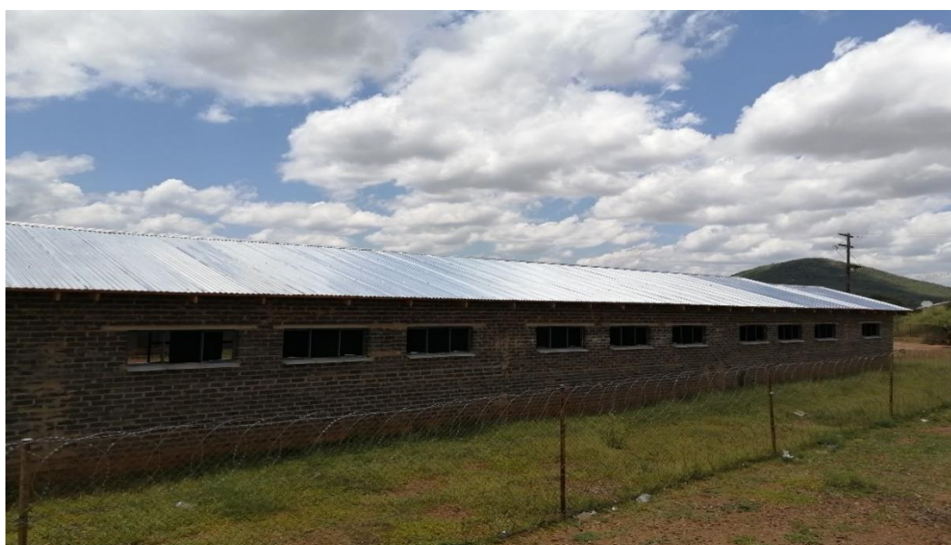
Figure 1: Newly constructed classrooms
