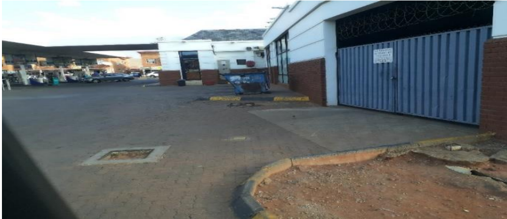
Figure 2: Engen Service Station in Kempton Park Commissioner Street
