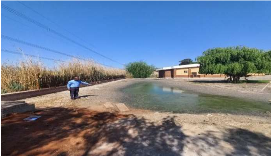
Picture 2: Sewage wastewater forming a pond at the church's back yard at 21 Pikkewyn Street.
