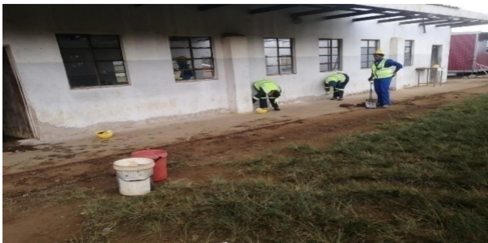
Figure 30: Progress at Mhlambansila
