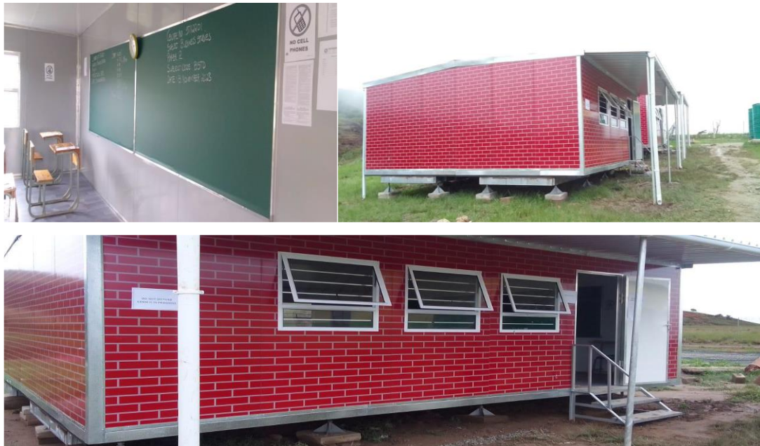
Figures 22: Mobile classrooms delivered at Bantubaningi
