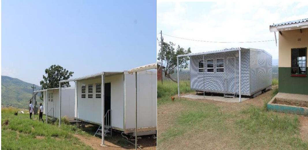
Figure 27: Three mobile classrooms delivered at Sizabonke
