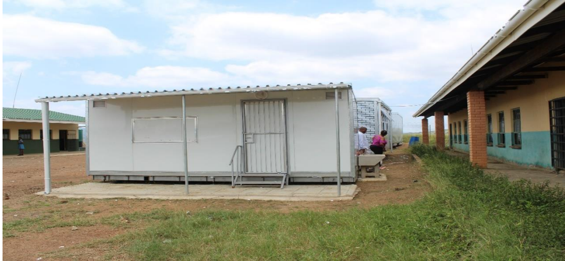
Figure 25: Mobile classrooms delivered at Zombode
