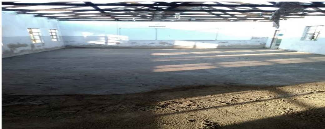
Figure 29: Progress at Mhlambansila
