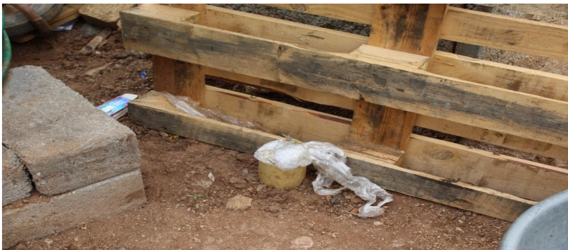
Picture 17: Pipe connected by a resident to direct raw sewage from his yard to the street
